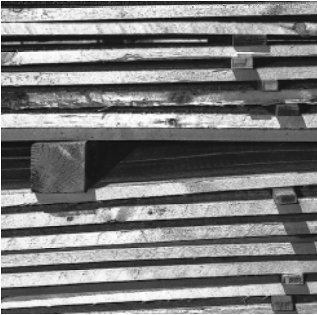
Figure 40—Improper bolster-sticker alignment will increase the defect of bow or warp.
