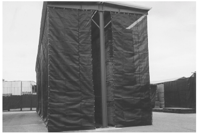
Figure 30—Shade cloth or any loose weave fabric can be used in air drying and shed drying to reduce degrade resulting from uncontrolled rapid drying and exposure to the sun and rewetting.
