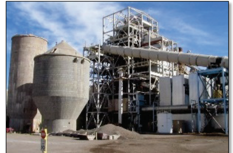
A biomass power plant that uses biomass from forest restoration as fuel.
